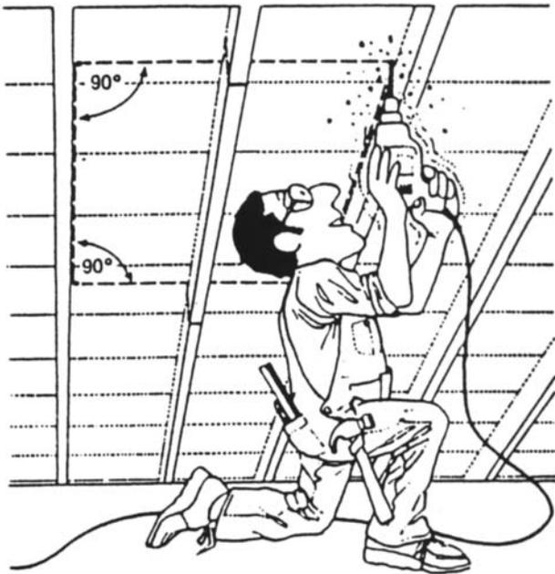
**1 Preparing an opening in the roof.** Opening should be positioned between rafters or trusses in accordance with desired day lighting effect. Drill holes through roof from inside at precise corners of the planned skylight opening, using **INSIDE** curb dimensions.
