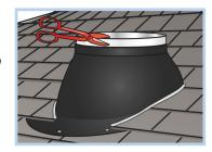
**STEP 13 -** Use a knife to score the protective film by cutting along the outside of the channel of the light pipe. Then peel off all of the protective plastic film from all areas of the light pipe.
